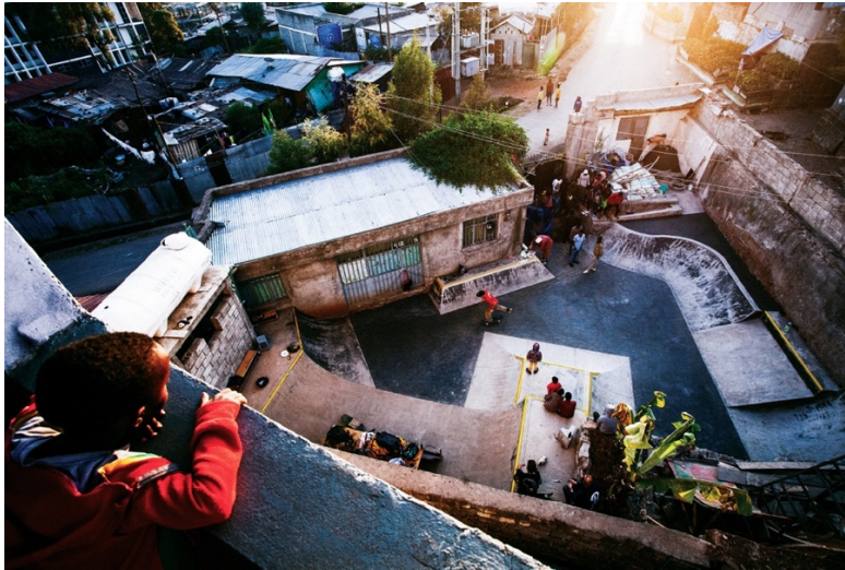
The morning after completion of the concrete work.
