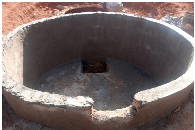
Figure 12: Plastering the biodigester
