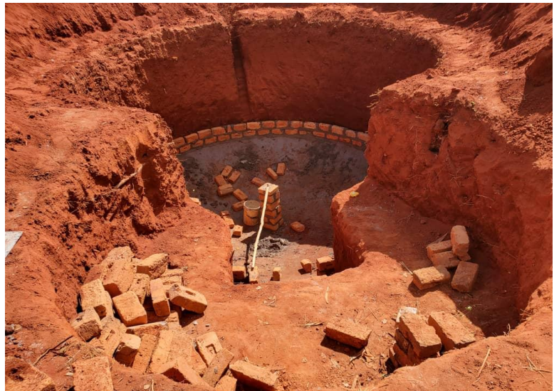
Figure 10. Concave base casting
