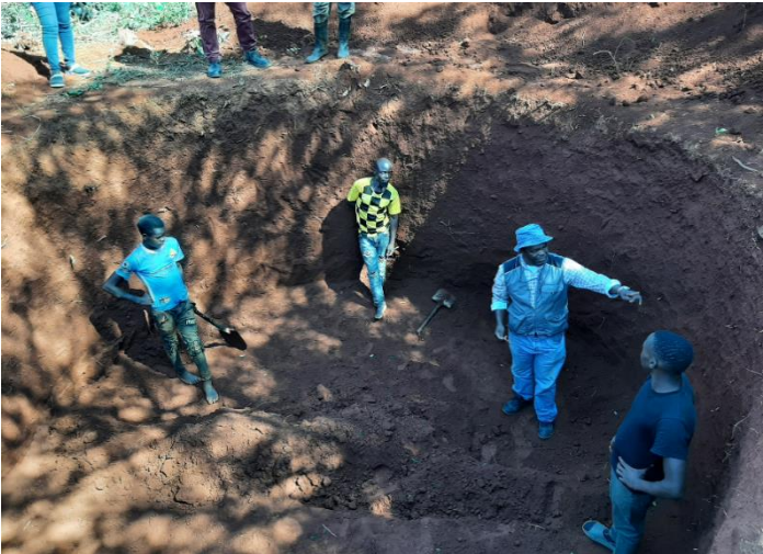
Figure 7. Inspecting the dome pit
