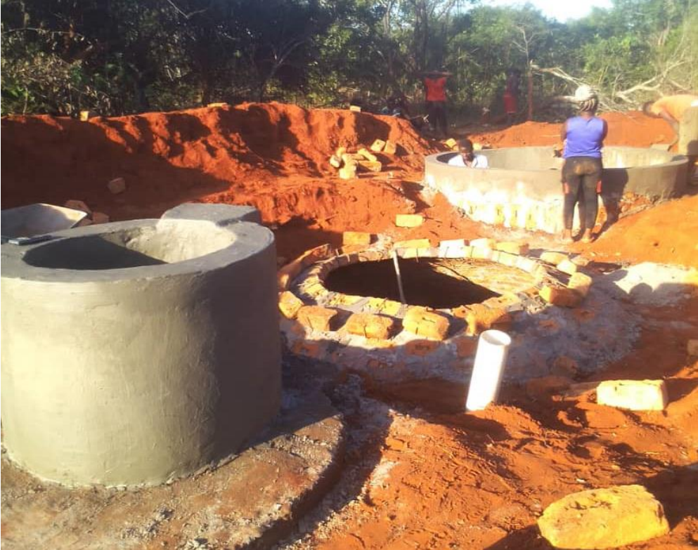
Figure 13. Final works on expansion chamber and gas outlet
